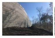
MSE Form Walls are often used for temporary and permanent applications in wetlands, detention ponds and shoreline repair.
