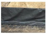
These geotextiles are primarily used to allow water to pass while keeping soil fines from migrating through the fabric.
